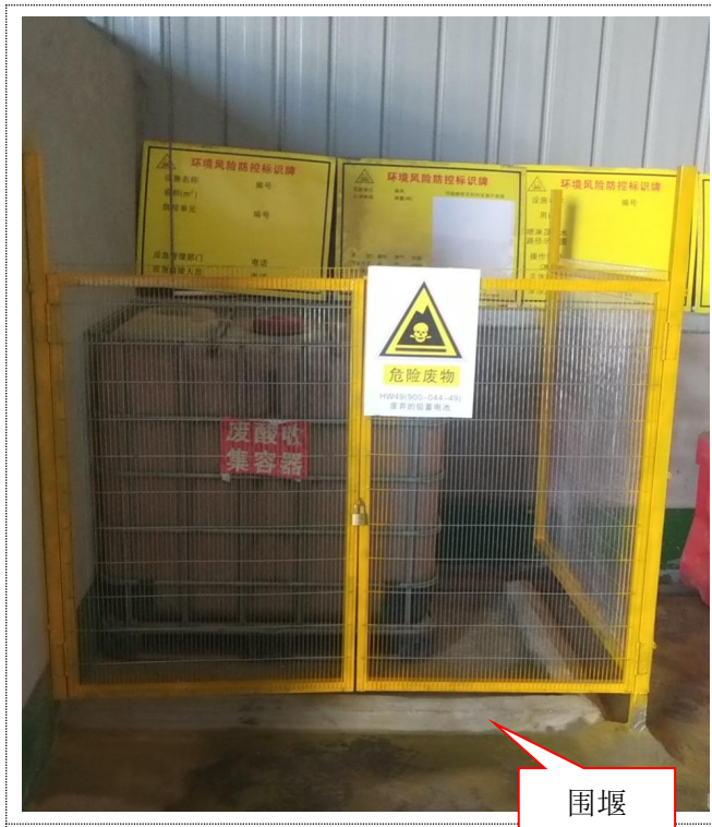
危废暂存区及标牌
